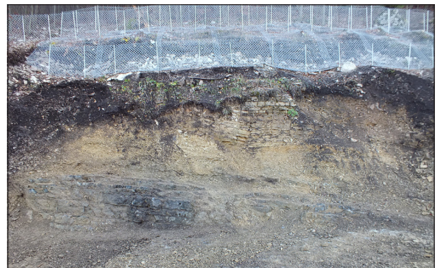
A protective mesh has been installed at the outcrop exposing the internationally renowned Permian-Triassic boundary
